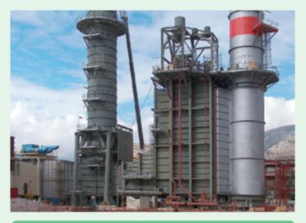
Baltec gas-turbine exhaust and heat recovery system
